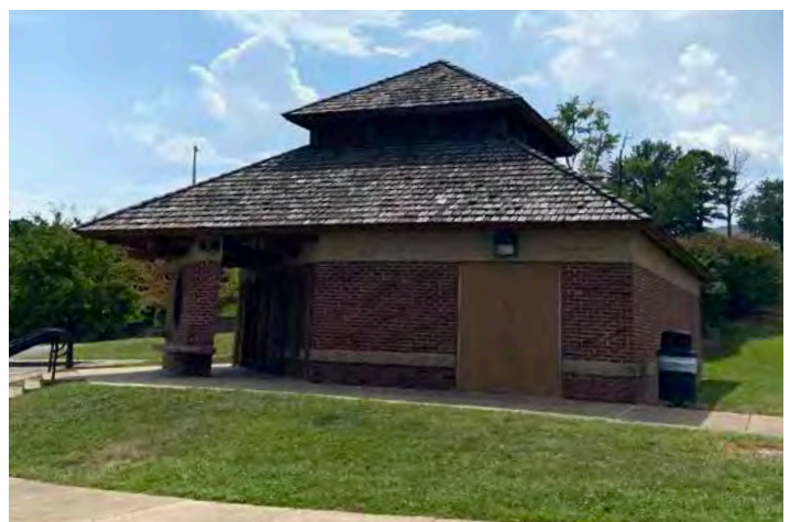
Figure 33: The larger restroom building adjacent to the parking area off Andrews Parkway.
