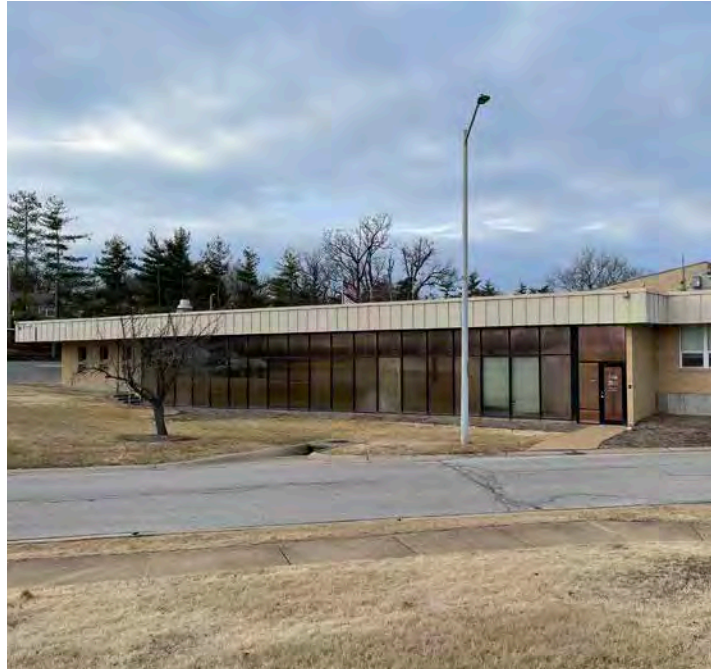
Figure 52: View of the current police station from the sand volleyball courts
