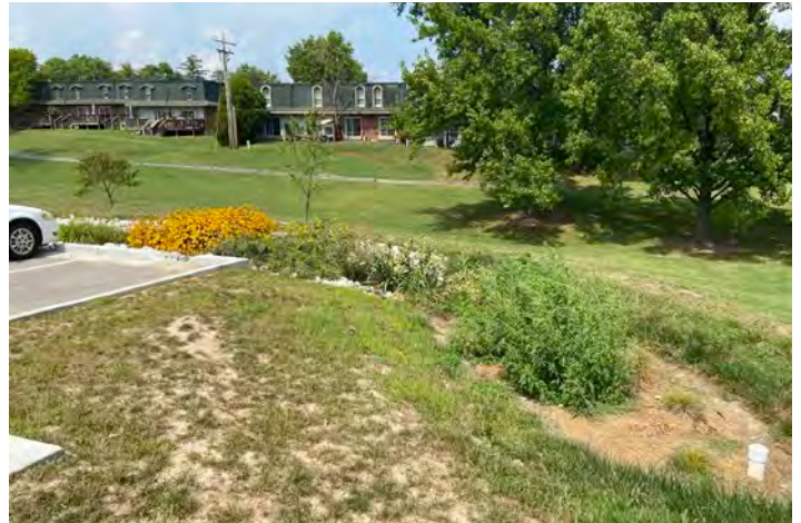
Figure 42: Bioretention cells help offset increased stormwater runoff created by impervious surfaces such as concrete or asphalt parking lots.
