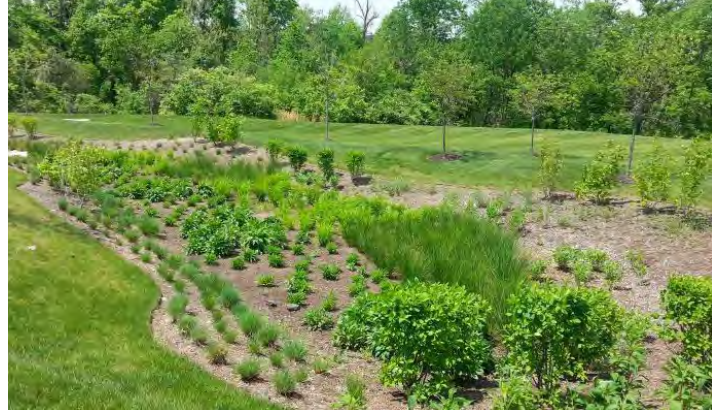
Figure 92: Newly planted bioretention basin used to mitigate stormwater runoff.
