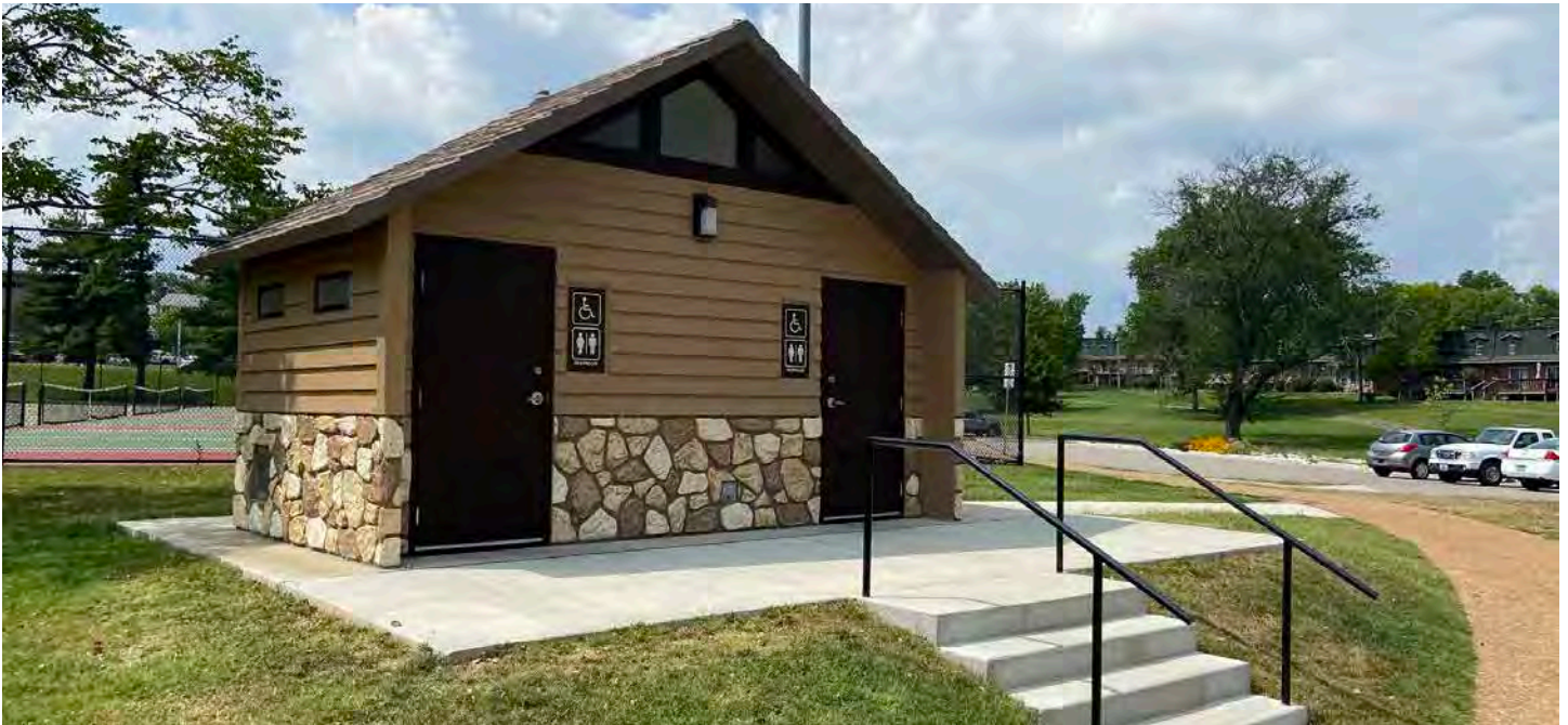
Figure 32: The new restroom facility provides easier access to park visitors utilizing the playground.
