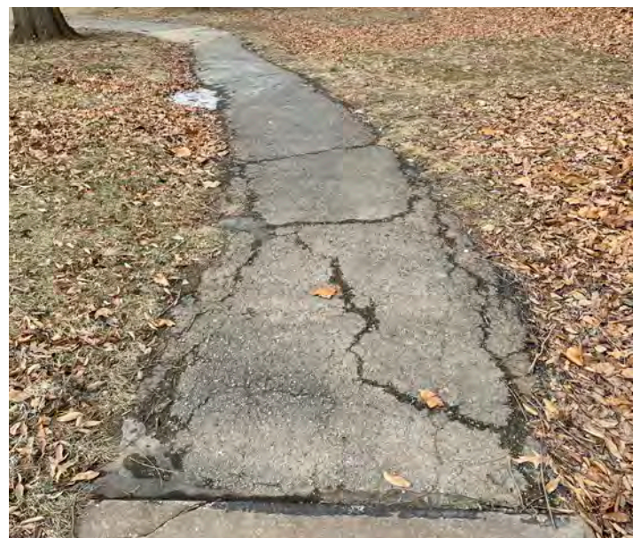
Figure 31: The asphalt path along the north side of the park creates a larger loop in the park but needs resurfacing.
