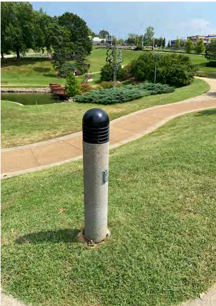
Figure 69: Light bollard with exposed aggregate finish.
