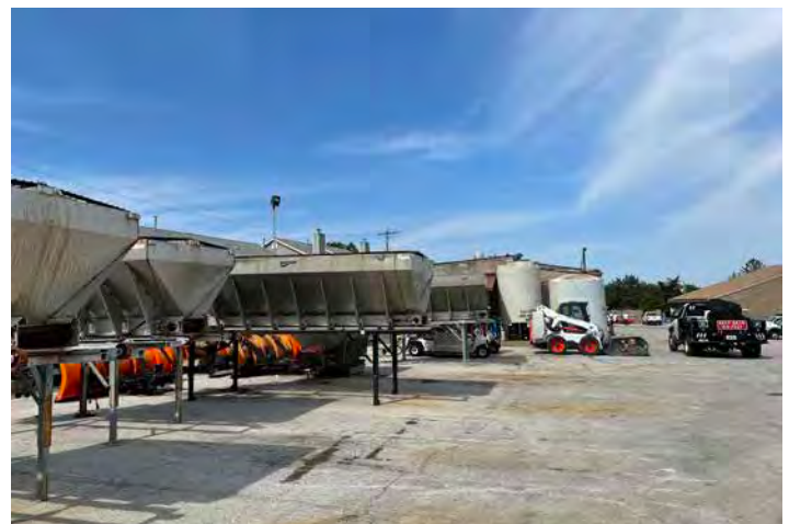
Figure 51: Much of the equipment and vehicles are too large to fit in the covered bays and are forced to be stored and serviced outside.
