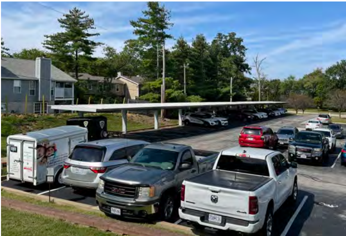
Figure 53: A portion of covered parking along the west property line
