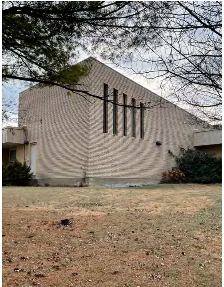
Figure 55: View of the current one story police station
